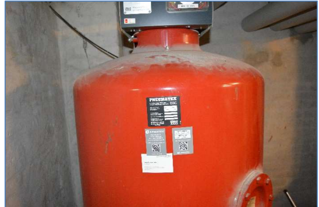
Foto 2: Trykexpansion - Trykholdestation
