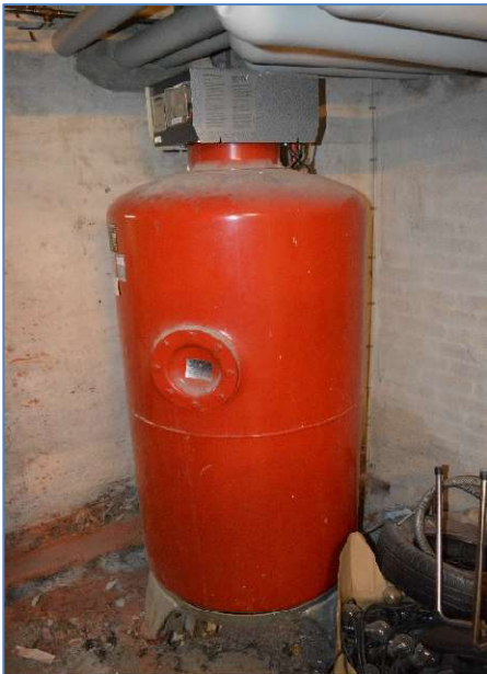
Foto 3: Trykexpansion - Trykholdestation
